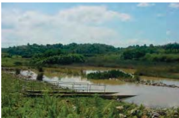
The condition of wetland cells
