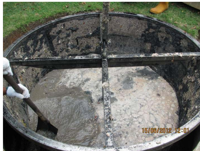
Refuse trapped in GPT in the process of being cleared out
