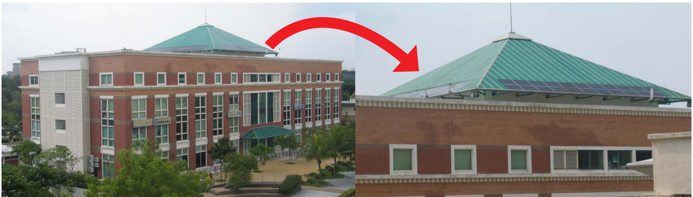
Danau Point office complex, Precinct 16.
