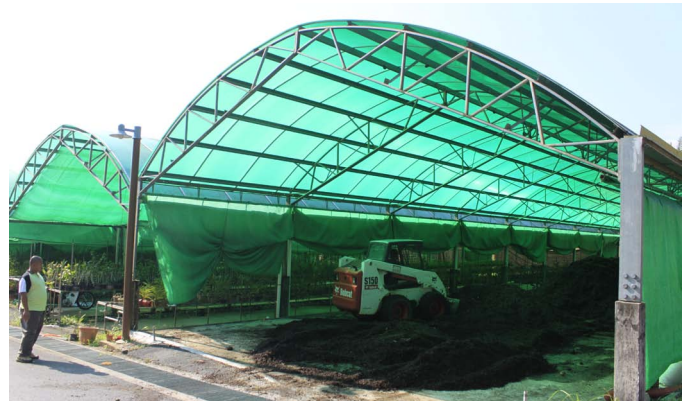
This tent can accommodate around 50-60 tons of compost.
