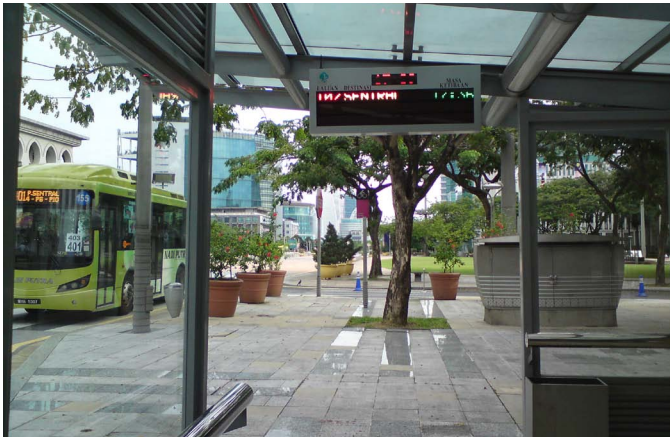
SVMS that has been installed at a bus stop near PJC Complex.
