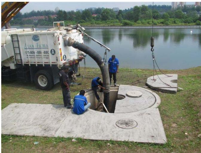
Refuse trapped in GPT in the process of being cleared out
