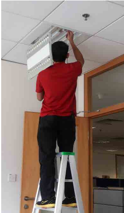
Installing energy saving lamps, brightness and movement detectors in the office.
