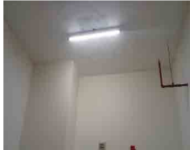
LED T8 Tube and T5 Fluorescent lamps at the stairways.
