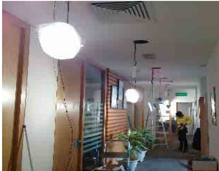
Installing energy saving lamps, brightness and movement detectors in the office.
