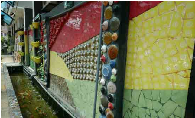
Corridor walls that are decorated with recycled items and fish pond that uses SPAH system
