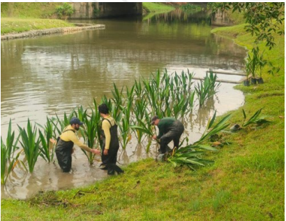
Aquatic plant replanting in wetland cells at Taman Wetland, Precinct 13
