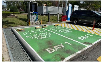
Installation of electric vehicle charging stations
