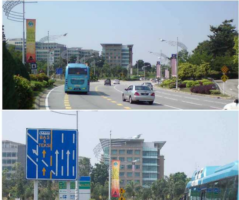
Dedicated bus and taxi routes marked with yellow lines and proper signage for other vehicles
