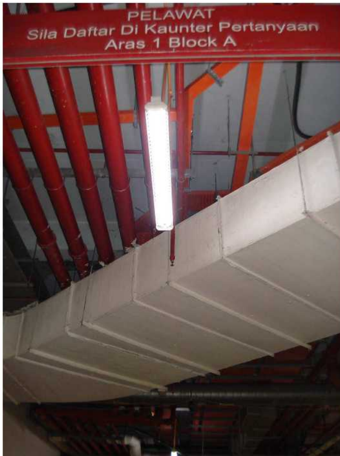
T6 lights as an alternative to LED as the cost is lesser.
