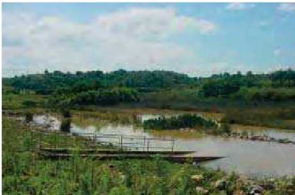
The condition of wetland cells
