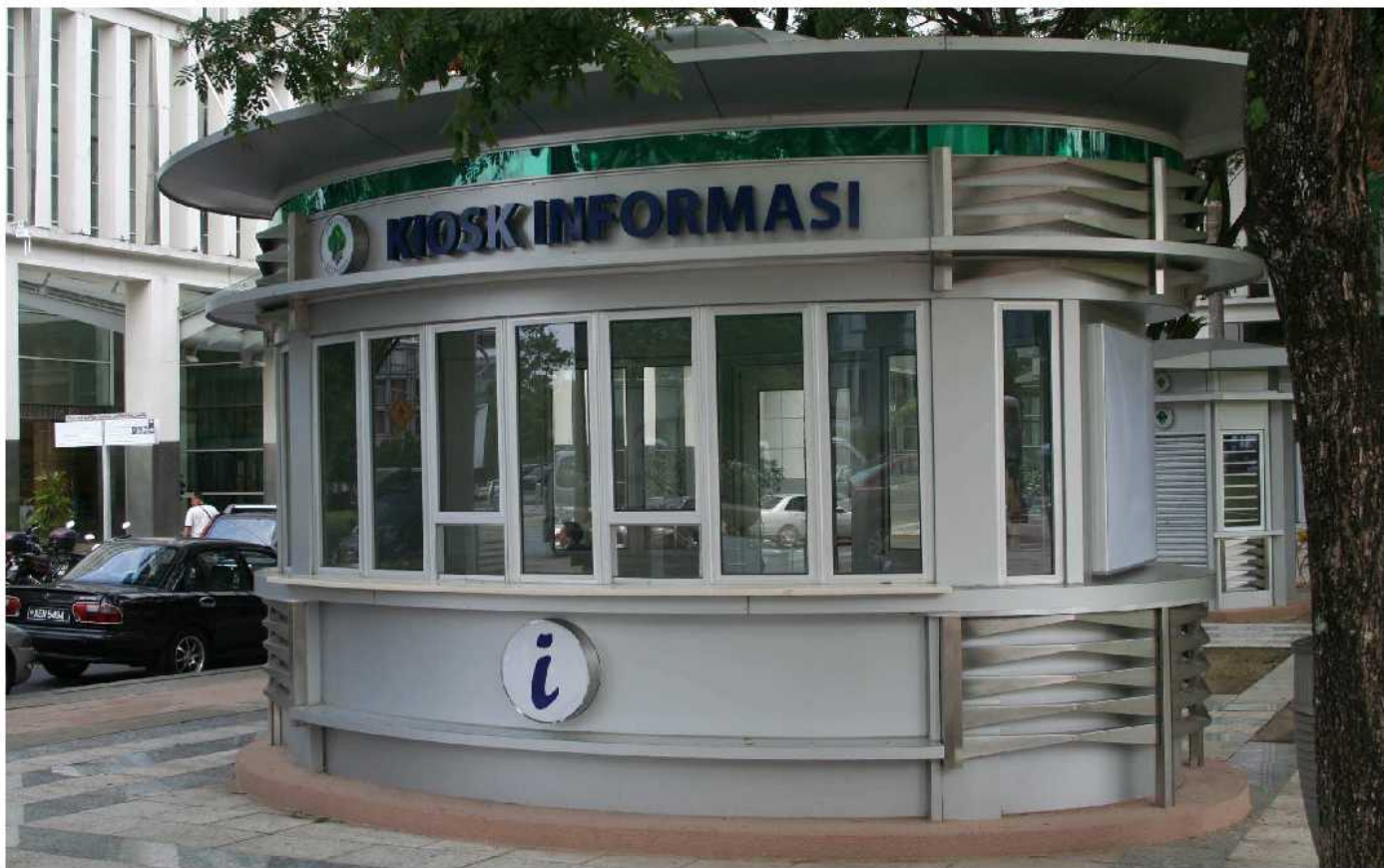
Small business kiosks near the PPJ complexes have been fitted with LED and T6 lights.
