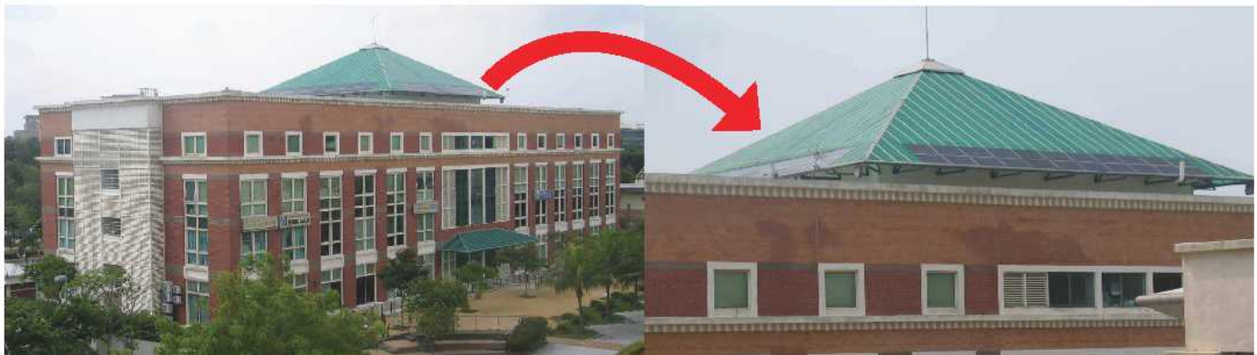
Danau Point office complex, Precinct 16.
