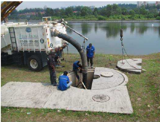
Refuse trapped in GPT in the process of being cleared out
