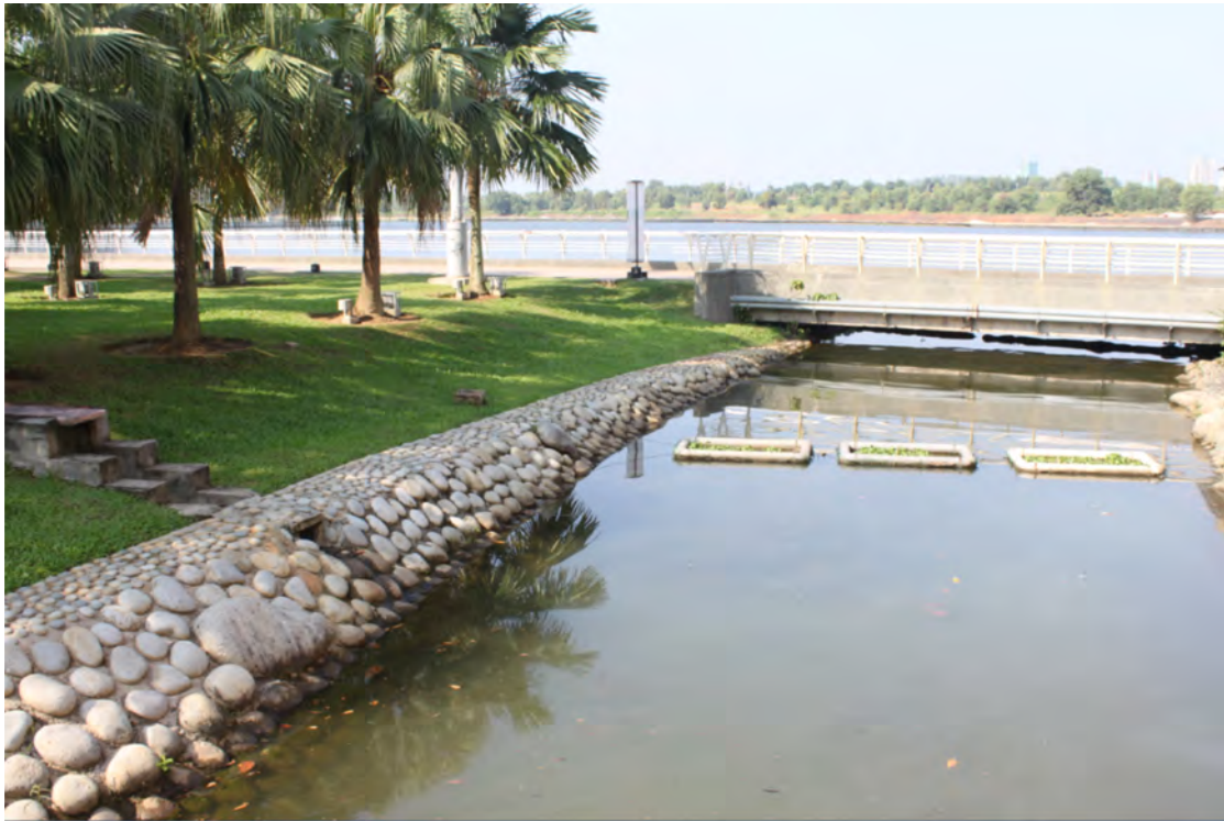
Floating aquatic plants is a method to treat discharge from drainage, before it enters into Putrajaya Lake.
