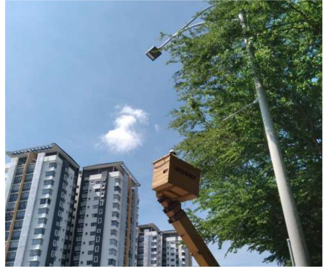
LED street light replacement works at Lebu Bestari, Precinct 16
