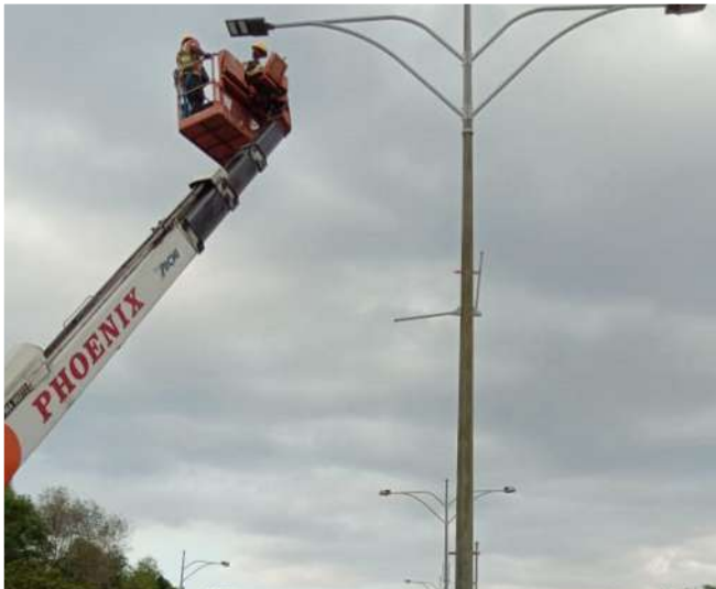
LED street light replacement works at Persiaran Timur
