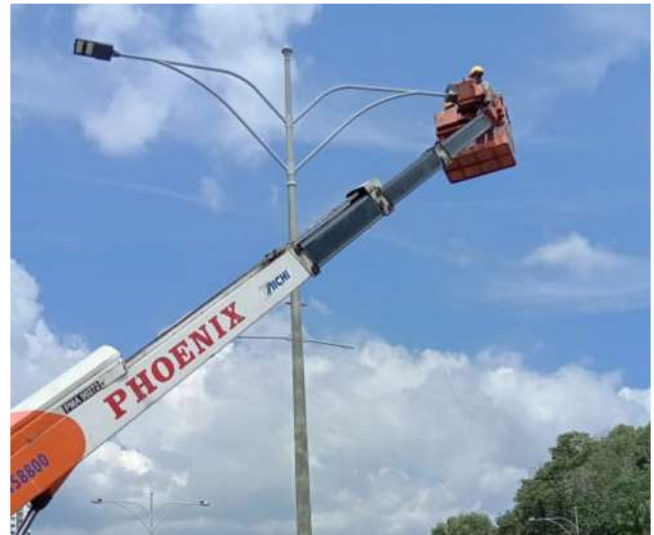
LED street light replacement works at Persiaran Timur
