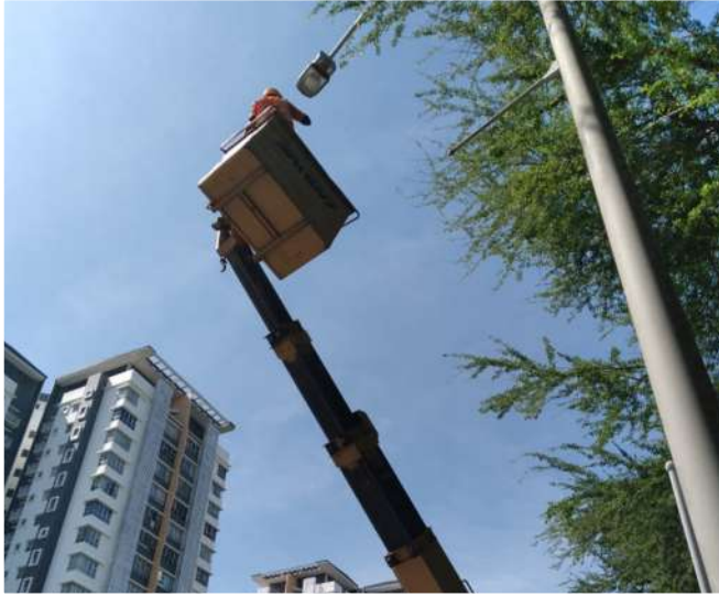
LED street light replacement works at Lebu Bestari, Precinct 16
