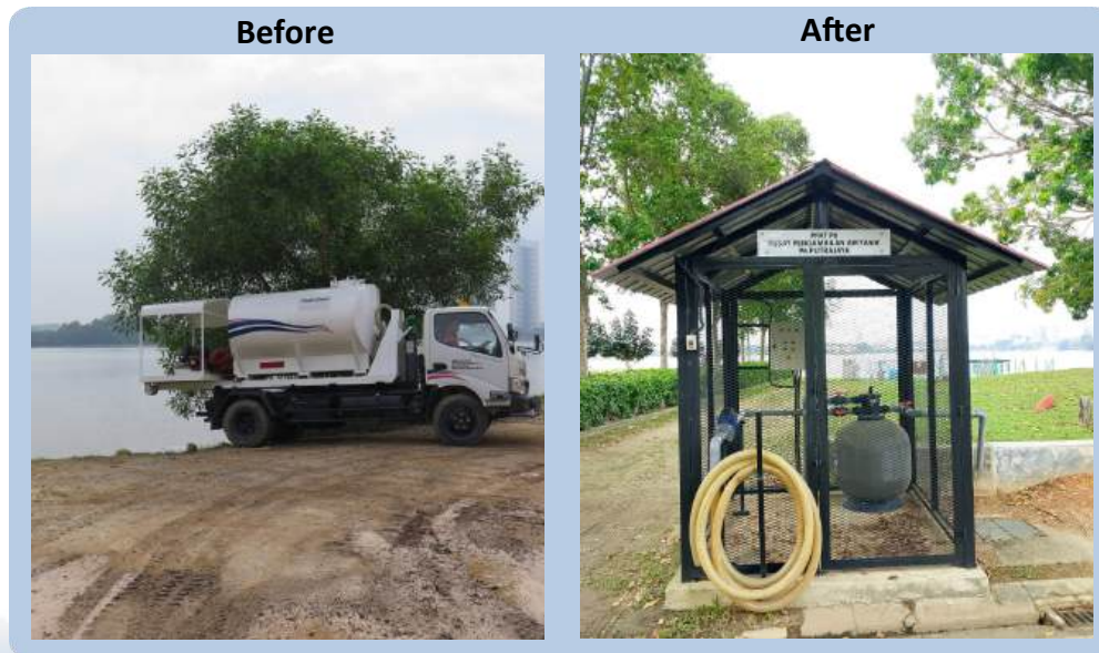
Lake water intake station, Precinct 6
