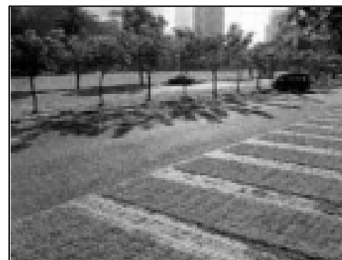
Figure 4.16 Pervious Surface for Parking Area
