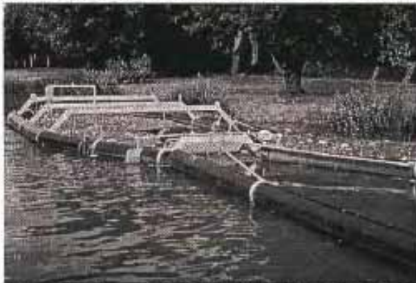
Figure 2.13 A floating litter trap placed on the receiving waters near a pipe outfall. (ref. Allison et al. , 1997)
