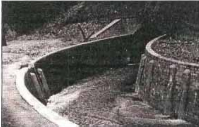
Figure 2.3 Urban waterways are often channelised and concreted to improve hydraulic efficiency
