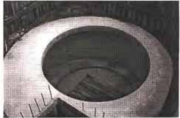
Figure 6.11 Shell of the chamber where the screens will be placed
