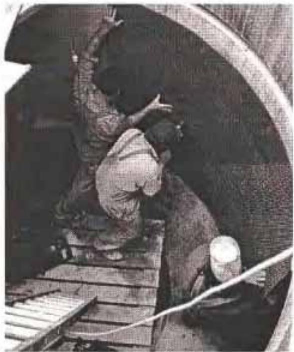
Figure 6.12 Fitting the separation screens.
