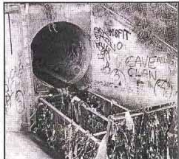
Figure 6.6 Litter Control Devices located at the pipe outfall (ref.Allison et al, 1997)
