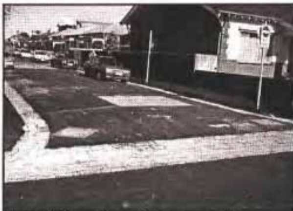
Figure 6.14 View of the completed construction at road level.
