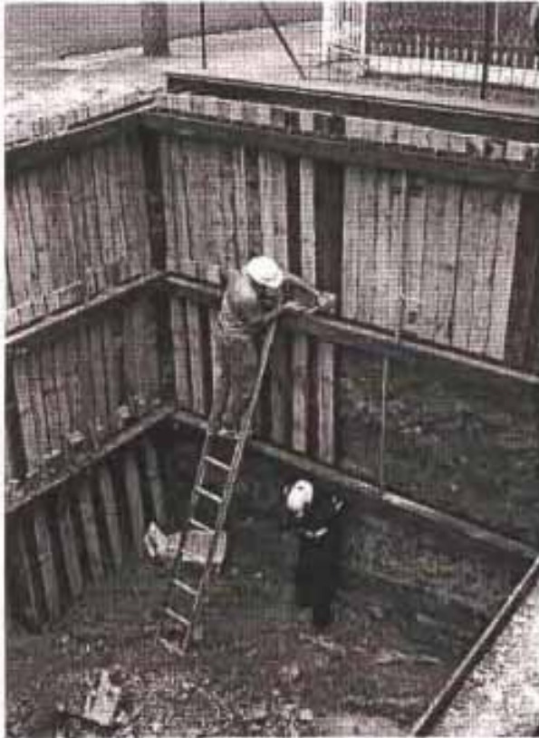
Figure 6.9 Excavation down to the floor of the chamber (6x6x4m).
