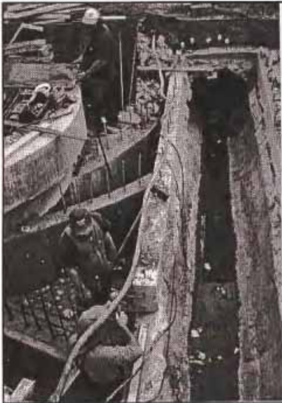
Figure 6.13 Breaking and connection to the adjacent to the stormwater pipe
