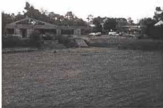
Figure 8.2 Playing field used as a Retarding Basin (Dry Detention Basin) Ref: Inst.of Engrs., Aust, 1987
