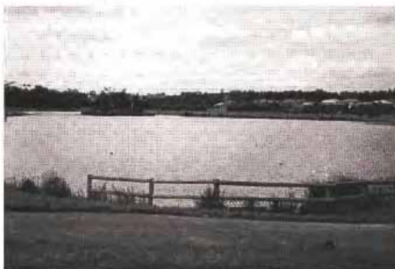
Figure 8.1 An urban pond used as a retarding basin (Wet Detention Basin)
