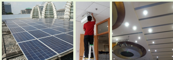
Installation of solar PV for selected government buildings
