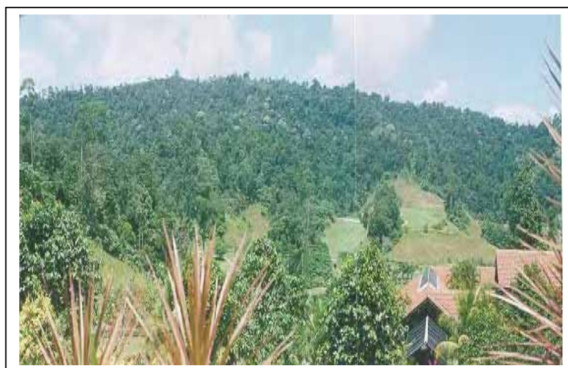
Figure 6.8 : Western part of West Country with proposed low density housing – Bungalow lots, located adjacent to IOI golf course.
