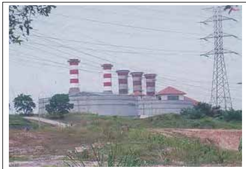
Figure 6.7: TNB Serdang Gas Turbine Power Plant
